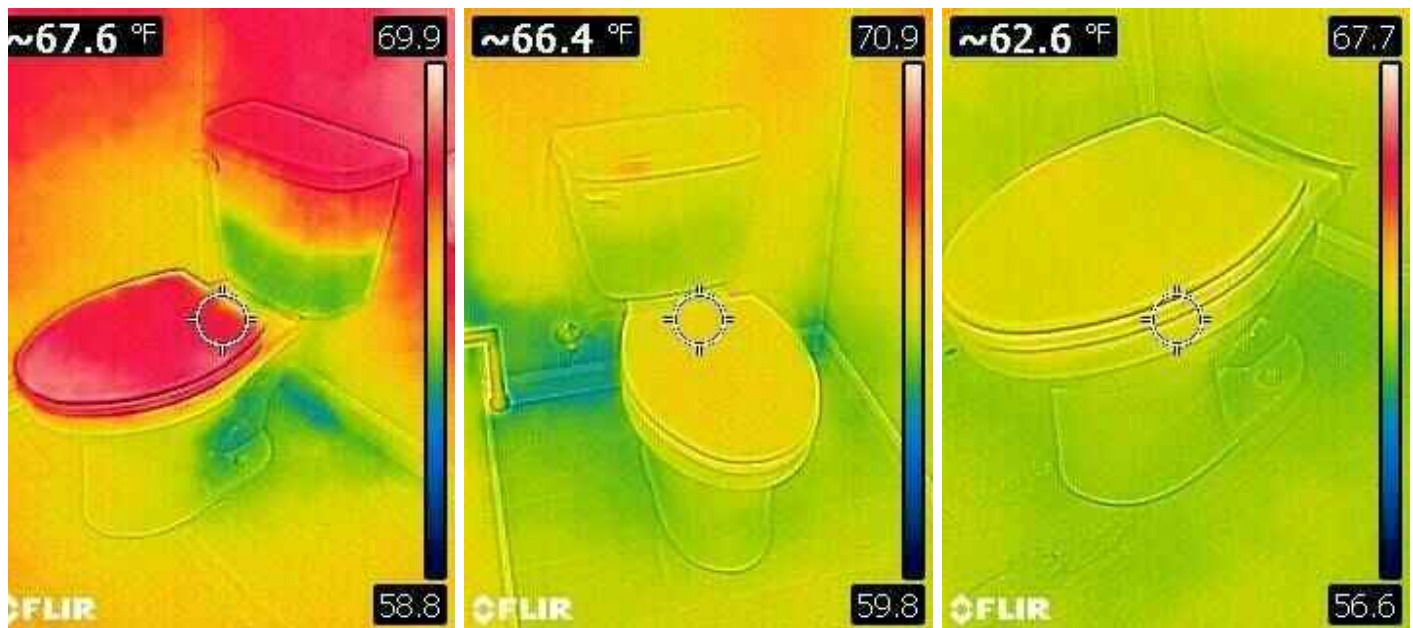
Thermal image scan for moisture leaks: Dry
