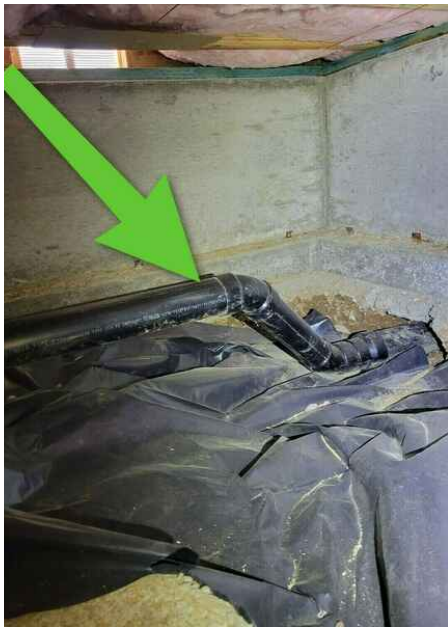
Main drain pipe. Southeast crawlspace.
