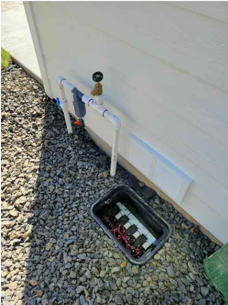
Exterior northeast corner.
