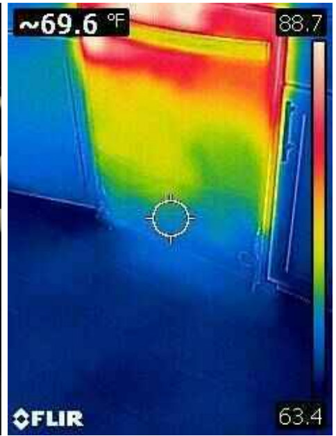
Thermal image scan for moisture leaks: Dry
