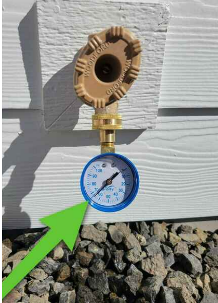
Water pressure tested ~68 psi.
