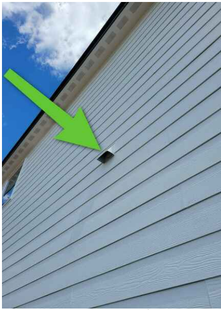
Exterior west side.
