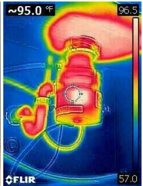
Thermal image scan for moisture leaks: Dry
